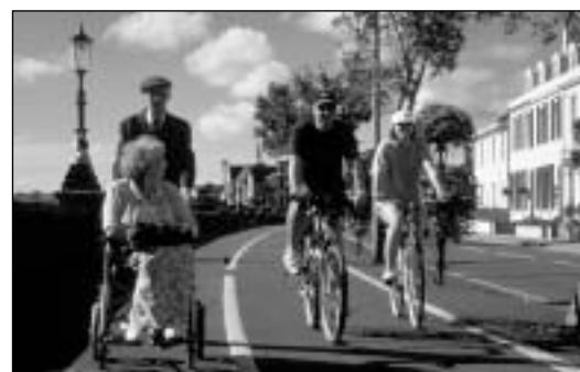
A previously pedestrian-only facility has been converted to shared use, with a raised tactile delimitation strip demarcating the pedestrians' and cyclists' sides. Barnstaple, Tarka Trail.
